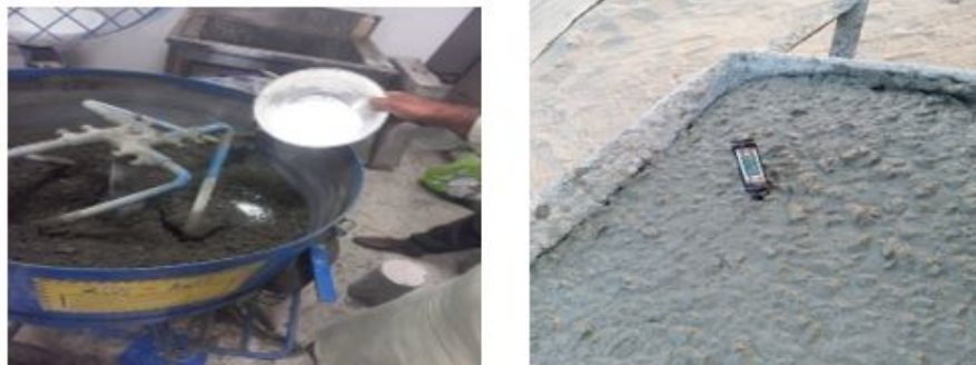
Figure 2: Mixing of concrete
